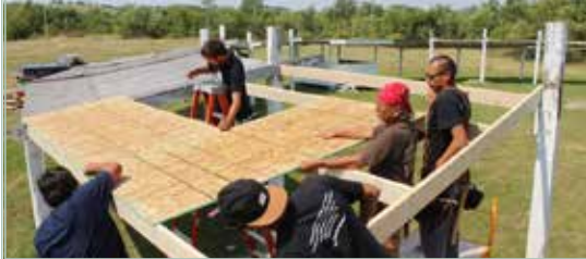
Working together on projects such as this repair of a shelter at local powwow grounds is part of the ethic encouraged by Thunder Valley.
