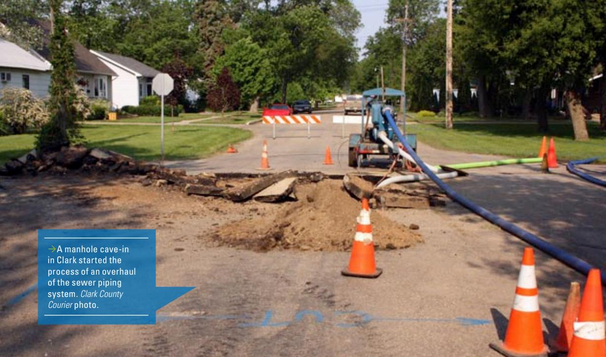
→ A manhole cave-in in Clark started the process of an overhaul of the sewer piping system. *Clark County Courier photo.*
